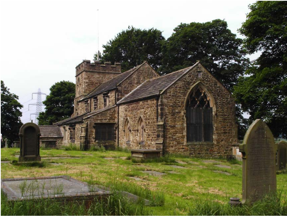
The church from the south east
