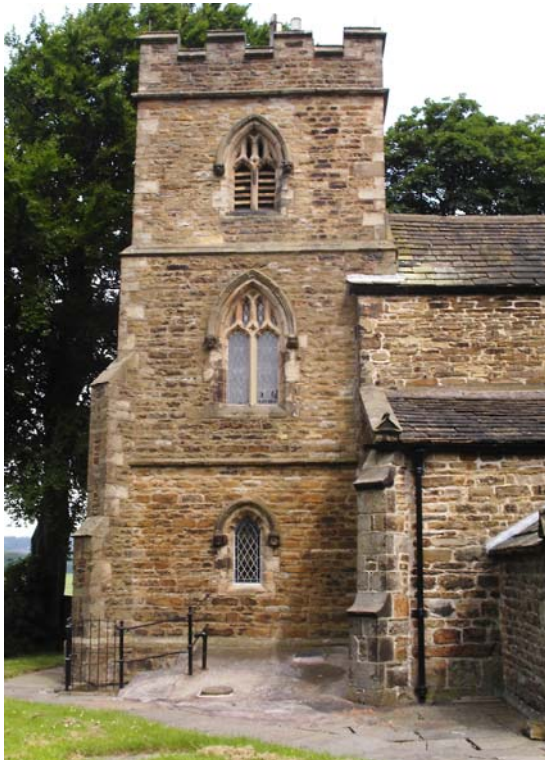
South elevation of tower
