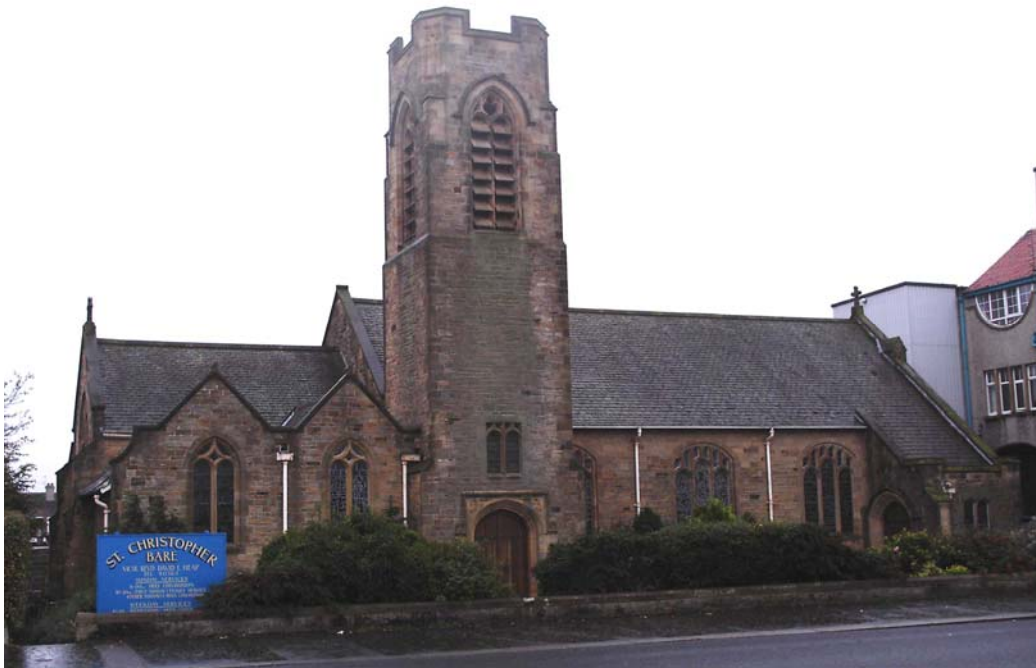
North view of Church
