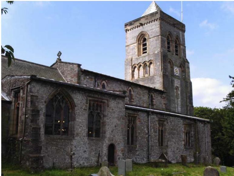
North west view
