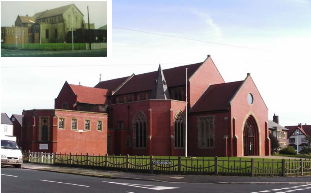
South west view of Church before and after Work of 2001
