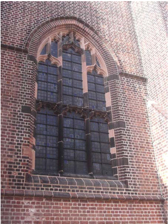
Detail of tower window terracotta repairs
