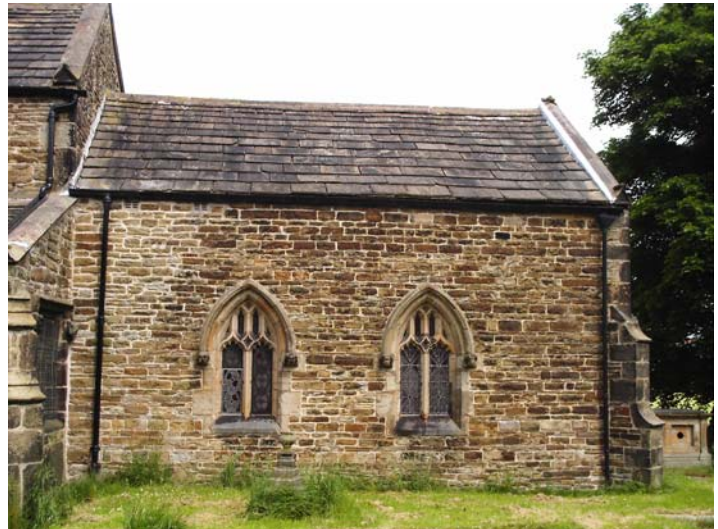
South elevation of chancel
