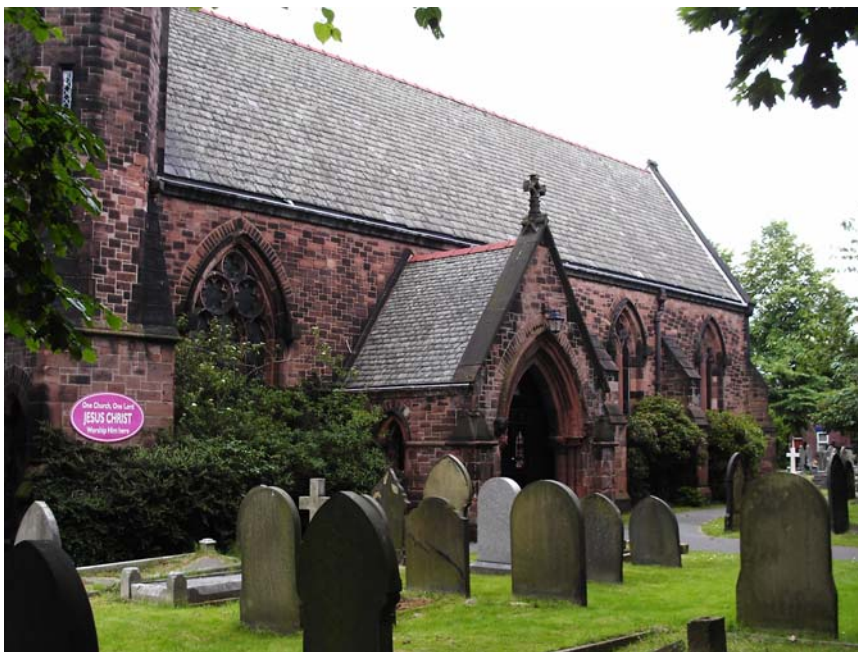
South porch and aisle
