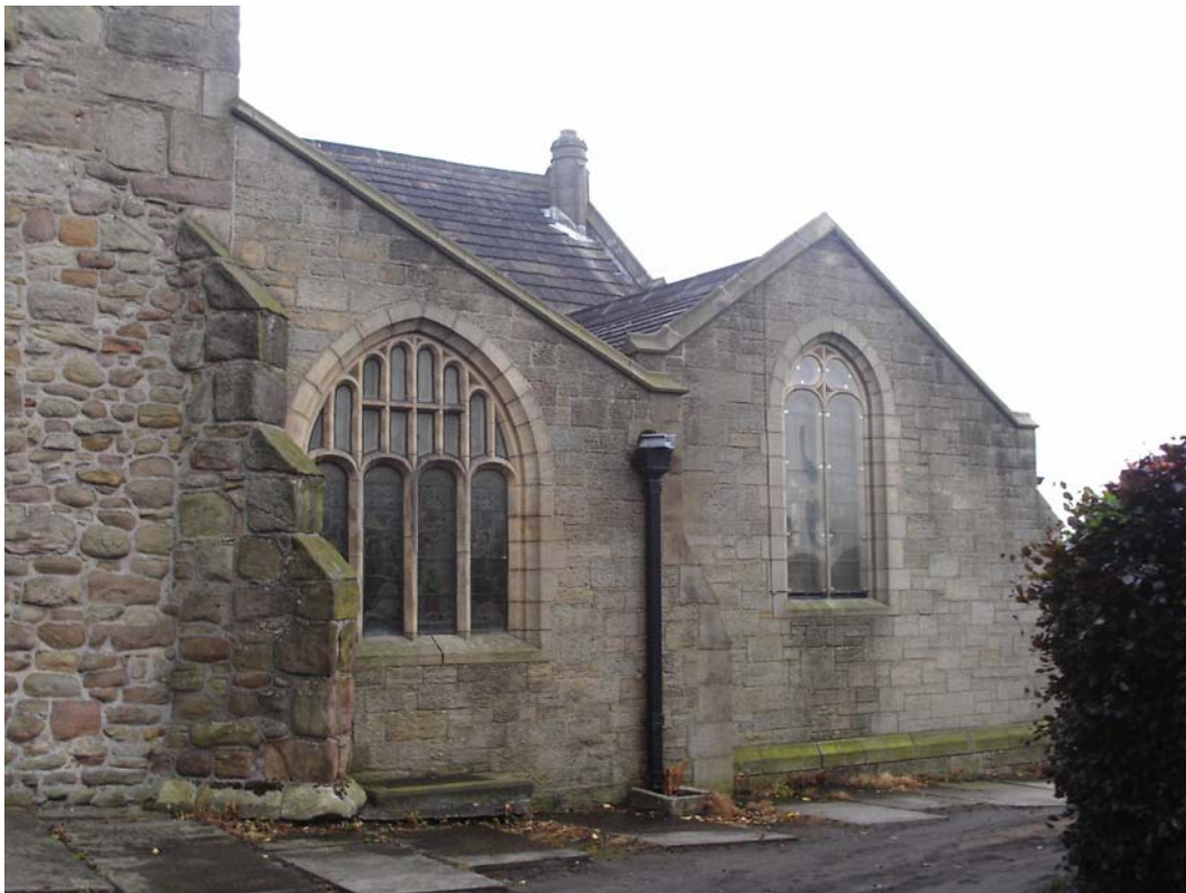
The east end of the north aisle
