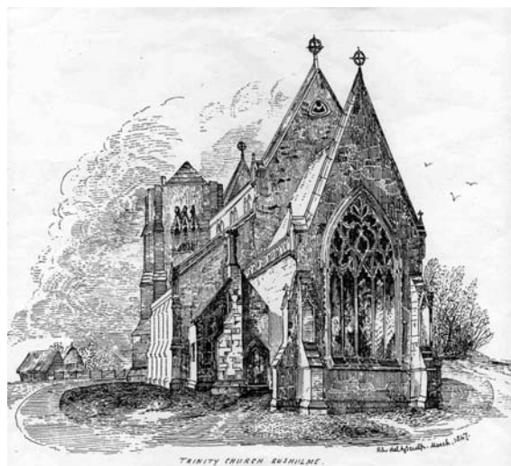
Fig. 5.20 The exterior from 1847 showing temporary roof
