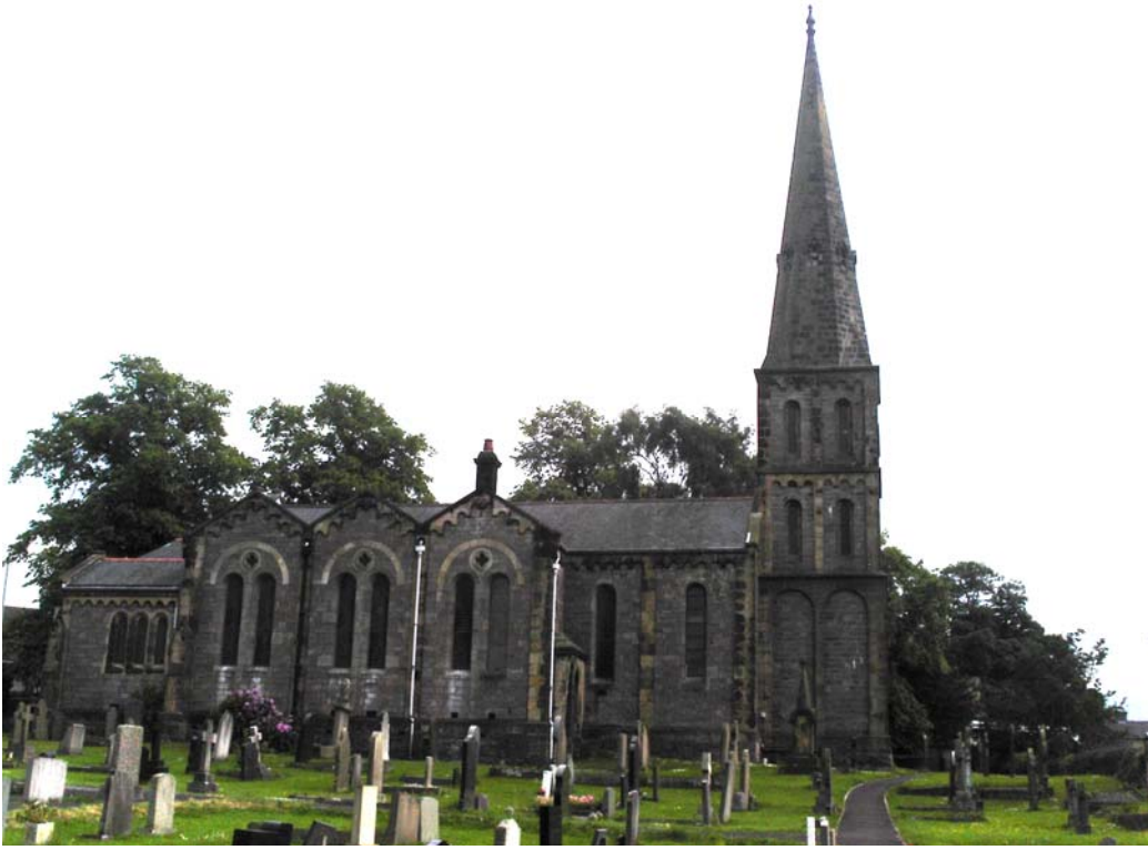
North view of Church
