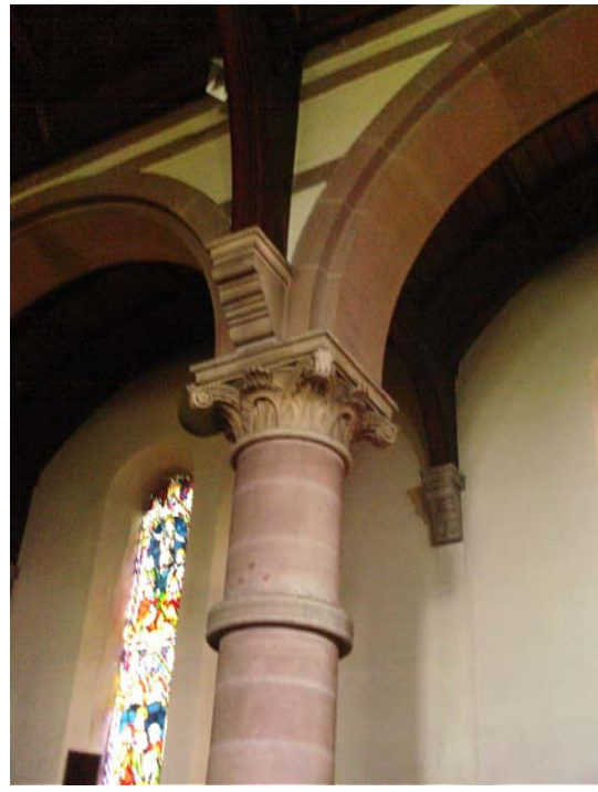
Detail of 1882 nave column
