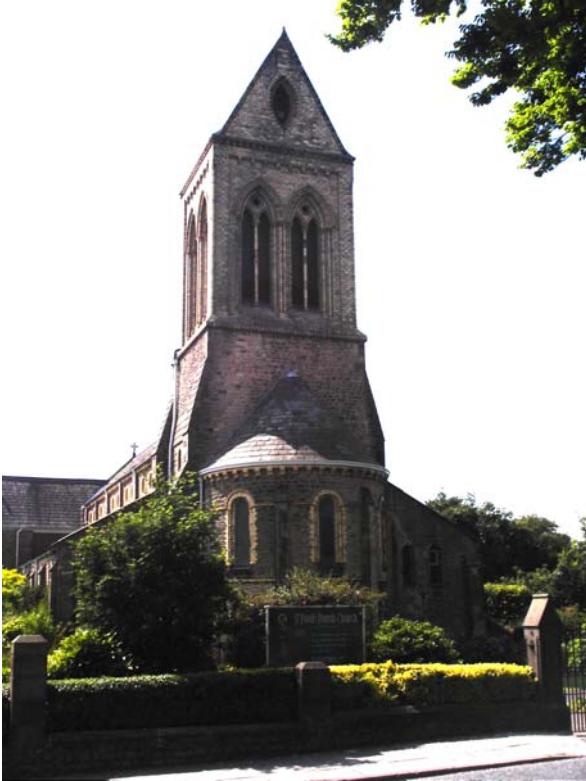
East view of Church
