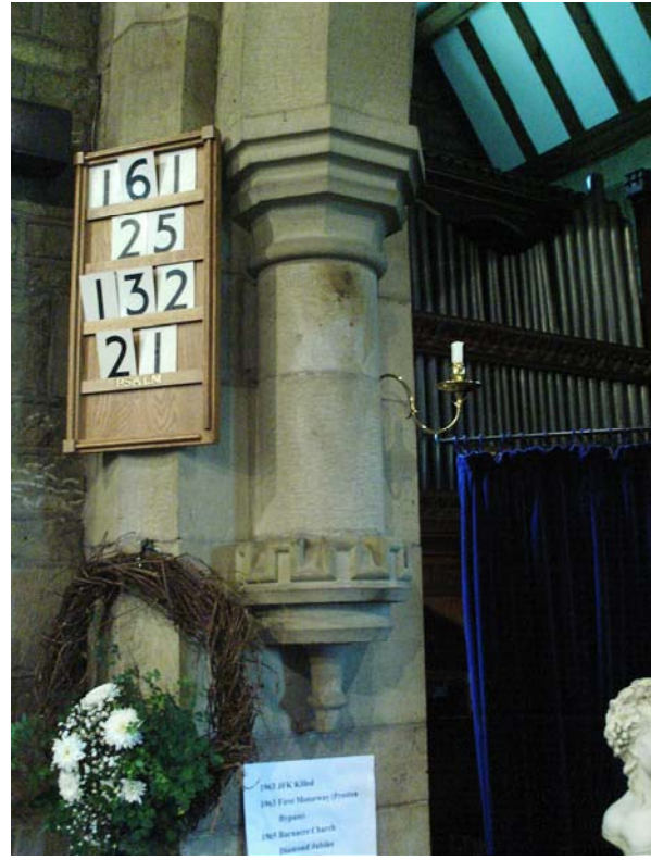
Detail of Chancel corbel
