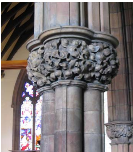
Fig. 5.19 Detail of column capital
