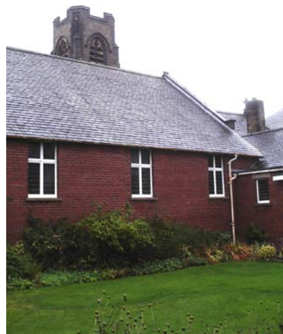
The incomplete south side
