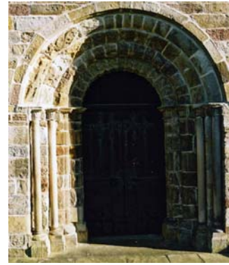
Fig. 9.3 Norman arch to tower
