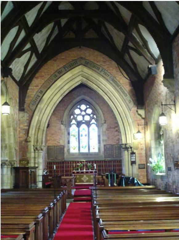
The interior facing east
