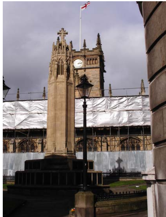
The scaffold over the north aisle
