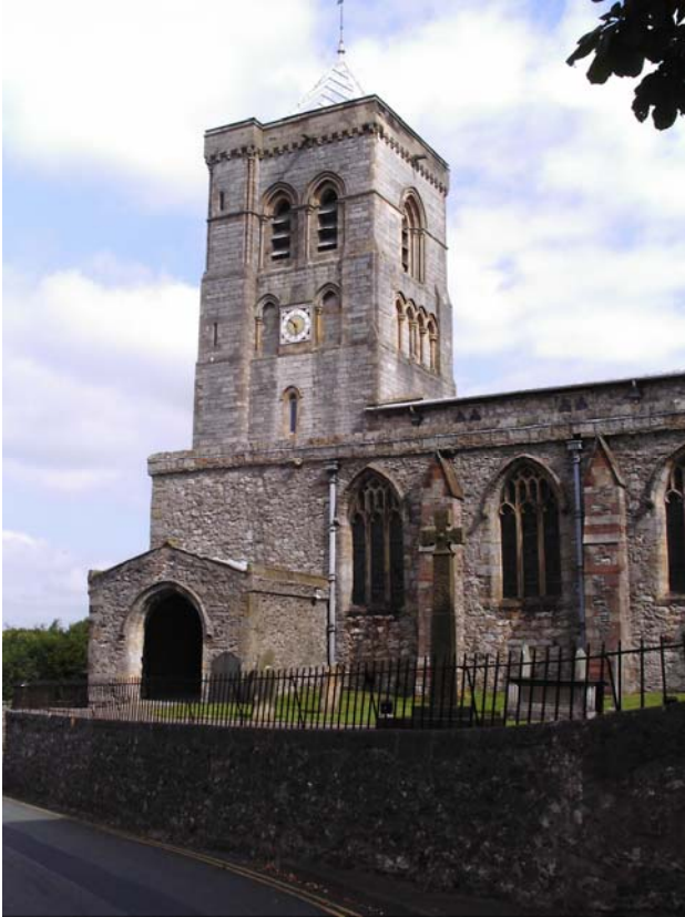
View of tower from south approach
