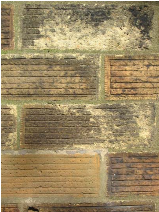
Detail of "masons tooling" note repair to bottom left
