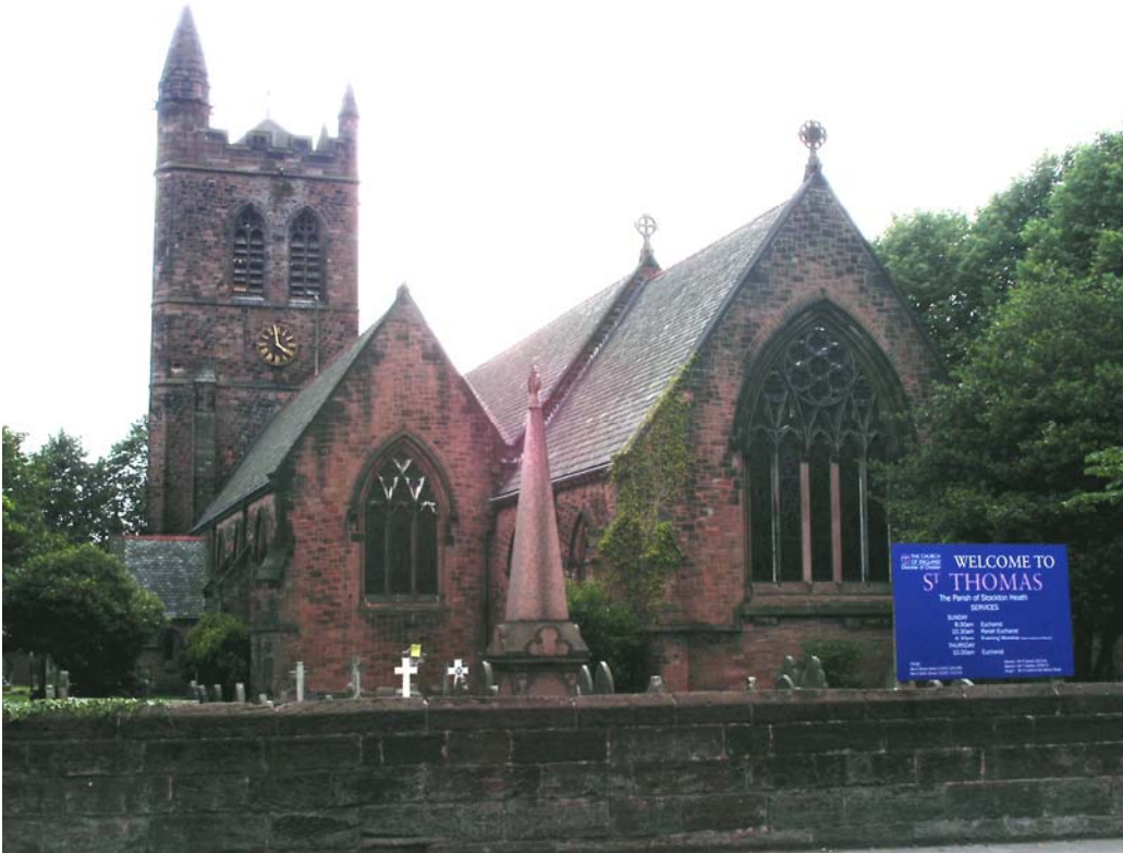
East view of Church
