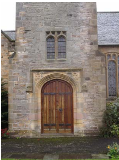
Detail of Tower Doorway
