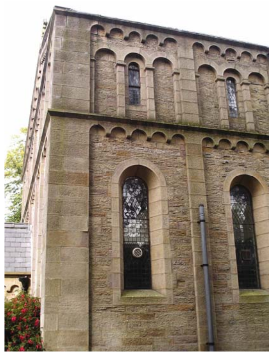
Detail of south side of nave
