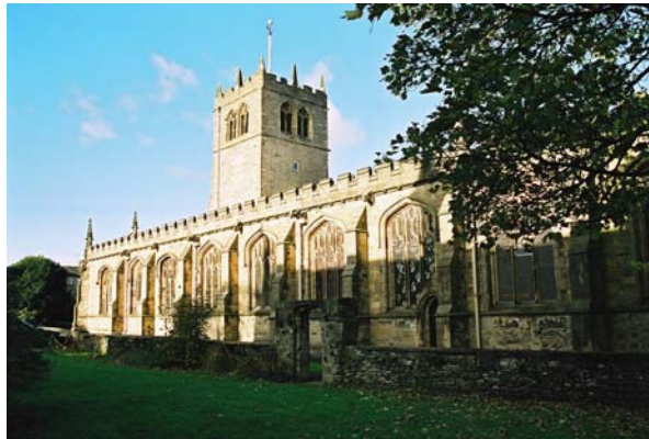
Fig. 9.2 Kendal Parish Church restored by J.S.Crowther in 1850's
