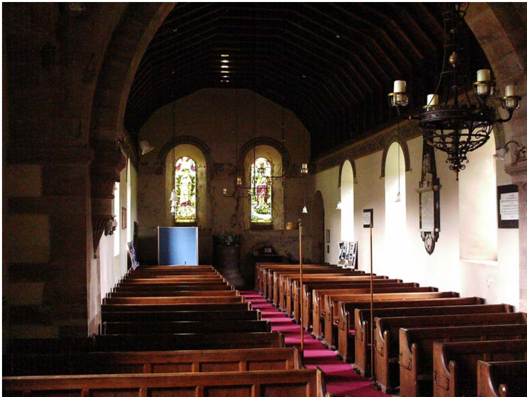
The Interior Facing West
