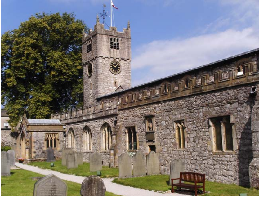
View of tower from south approach
