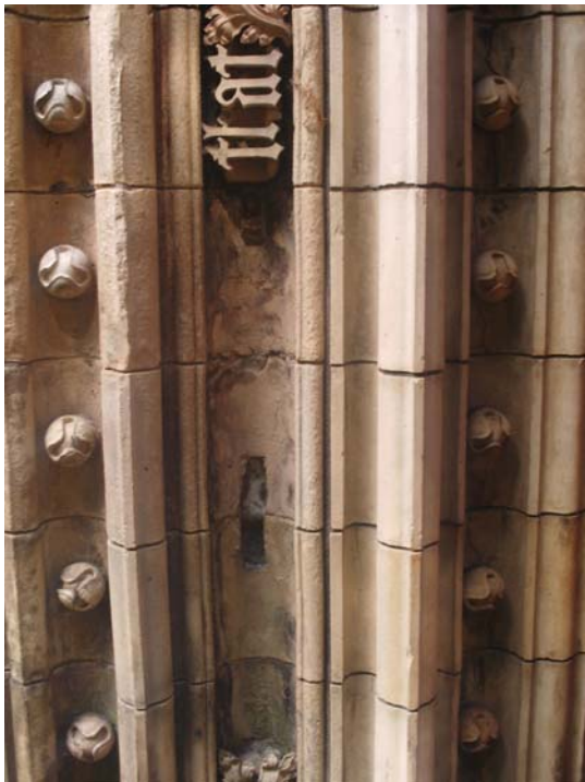
Detail of west door jamb
