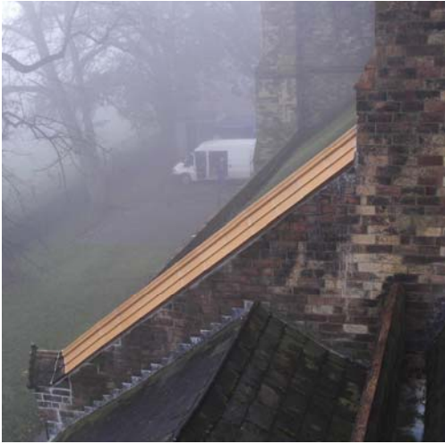
Fig. 5.23 The new terracotta copings
