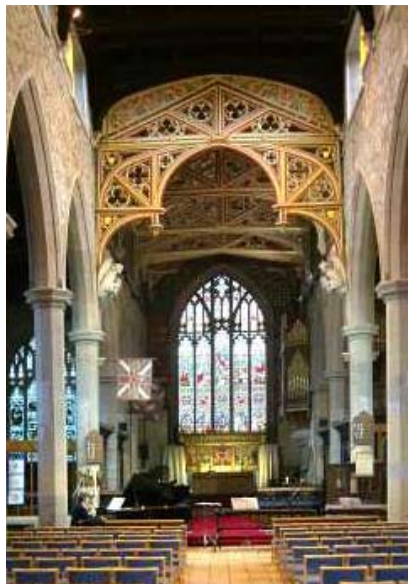
Fig. 9.8 The interior of St Peter's, Burnley note E.G.Paley's chancel arch
